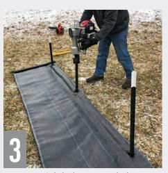
Start T-posts in holes between sand tubes (studded side facing fill slope), with the white end facing up. Set with a driver, pounder or sledgehammer.
