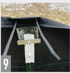
Tighten zip ties. The fabric will not be tight horizontally or vertically to allow the self-supporting curve to function.
