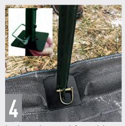
Drop bottom plate over end of post and place retainer clip on top. Finish driving T-post until bottom plate is tight and flush with ground, sealing tube pockets in place.
